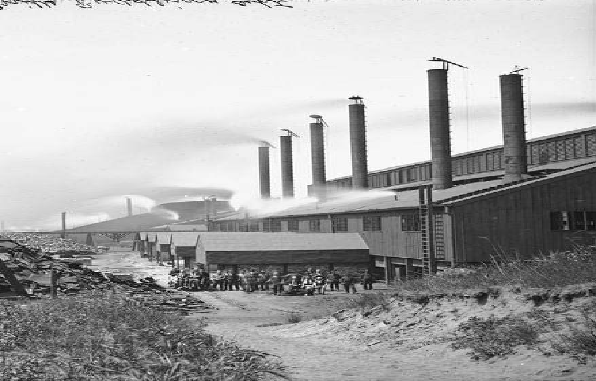
Bay View Rolling Mill, Shore of Lake Michigan, Milwaukee
