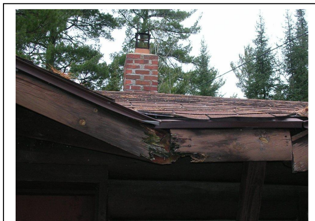
Figure 2-1. Roof Damage Example
