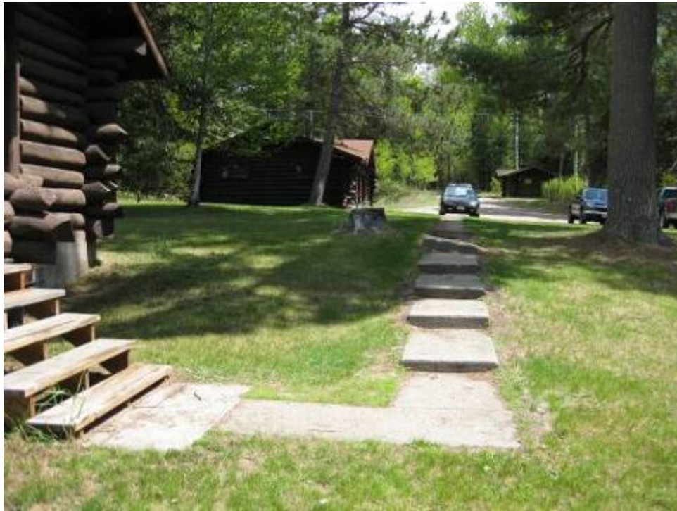
Figure 14. Concrete walkway connecting the main drive to the Ranger Dwelling is a contributing feature. (J. Ferguson: June 2, 2009)
