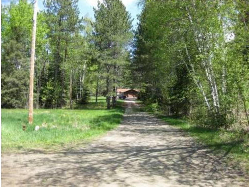
Figure 5. Primary road accessing the LSFES portion of the District has retained a preponderance of integrity and is considered a contributing feature of the historic district. (J. Ferguson: June 2, 2009)
