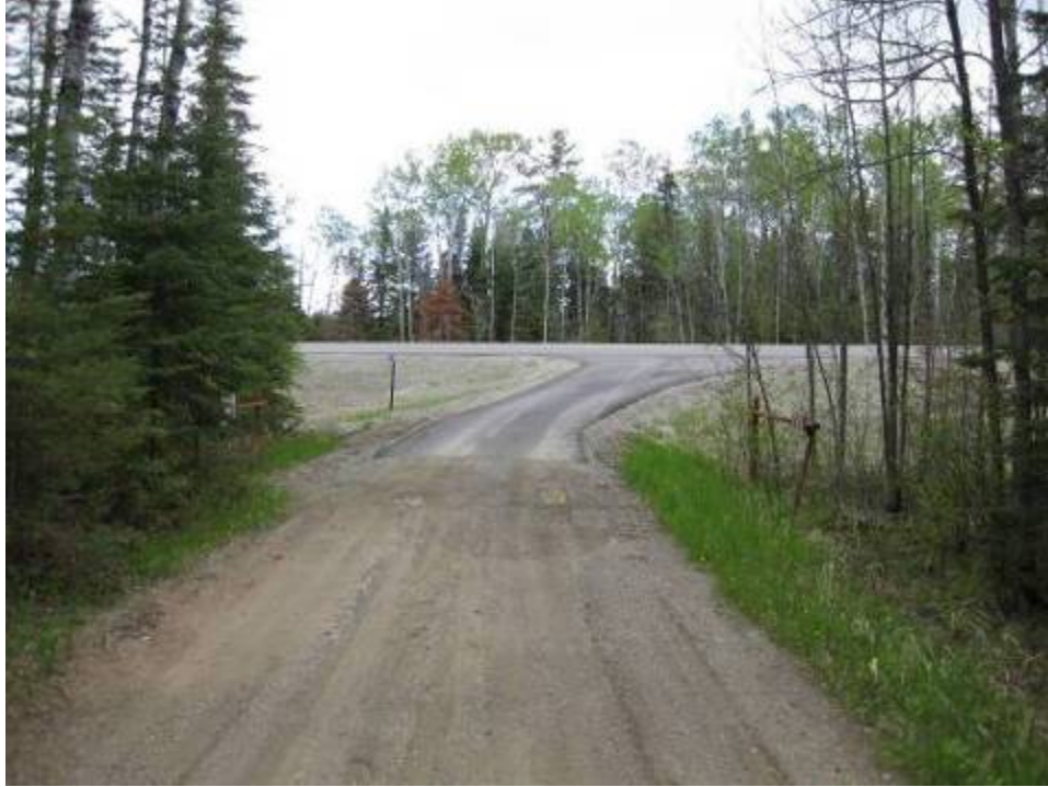
Figure 9. Southernmost entrance from HWY 1 has been altered due to road construction and is considered a non-contributing feature of the historic district. (J. Ferguson: June 2, 2009)
