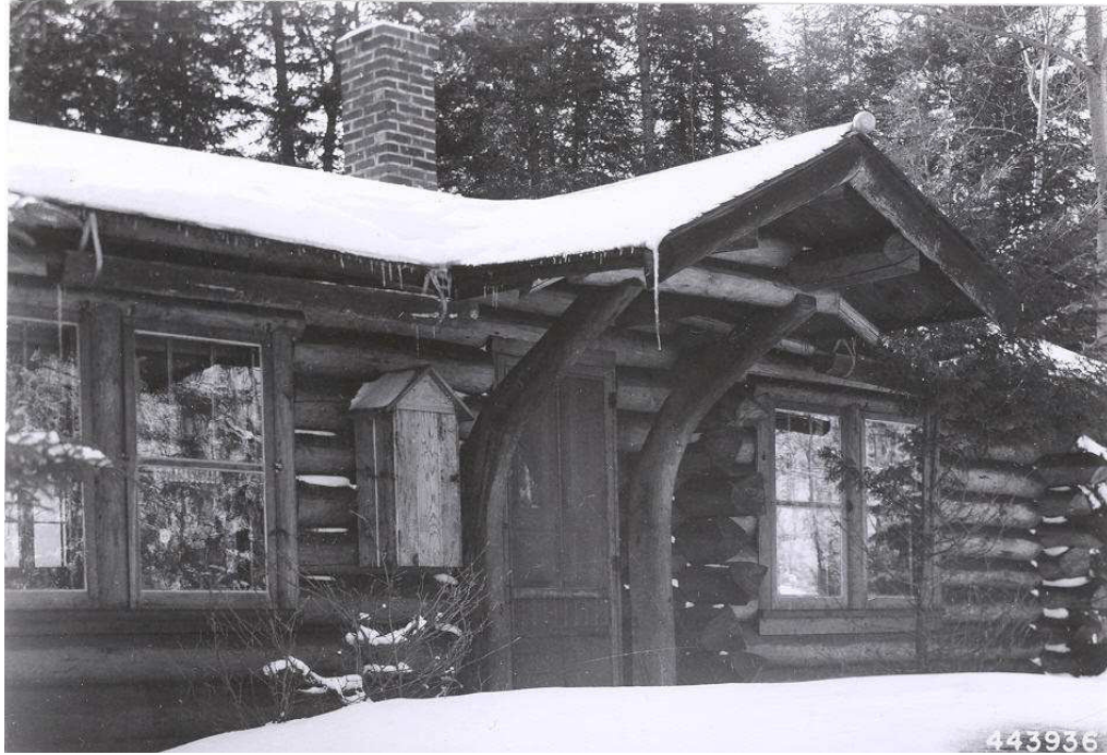
Figure 20. Front (northwest) view of the District Office building in 1947. View is from the north-northwest. Note the curved log brackets supporting the porch roof and hanging half-log gutters. (Photo courtesy of Superior National Forest).
