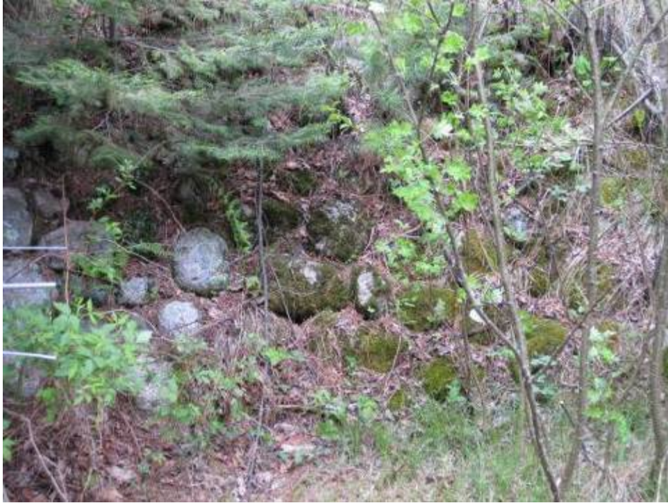
Figure 15. Stone retaining wall located between the Warehouse/Garage (FS Bldg. #31106) and the Cellar (FS Bldg. #31103) is a contributing feature. (J. Ferguson: June 2, 2009)
