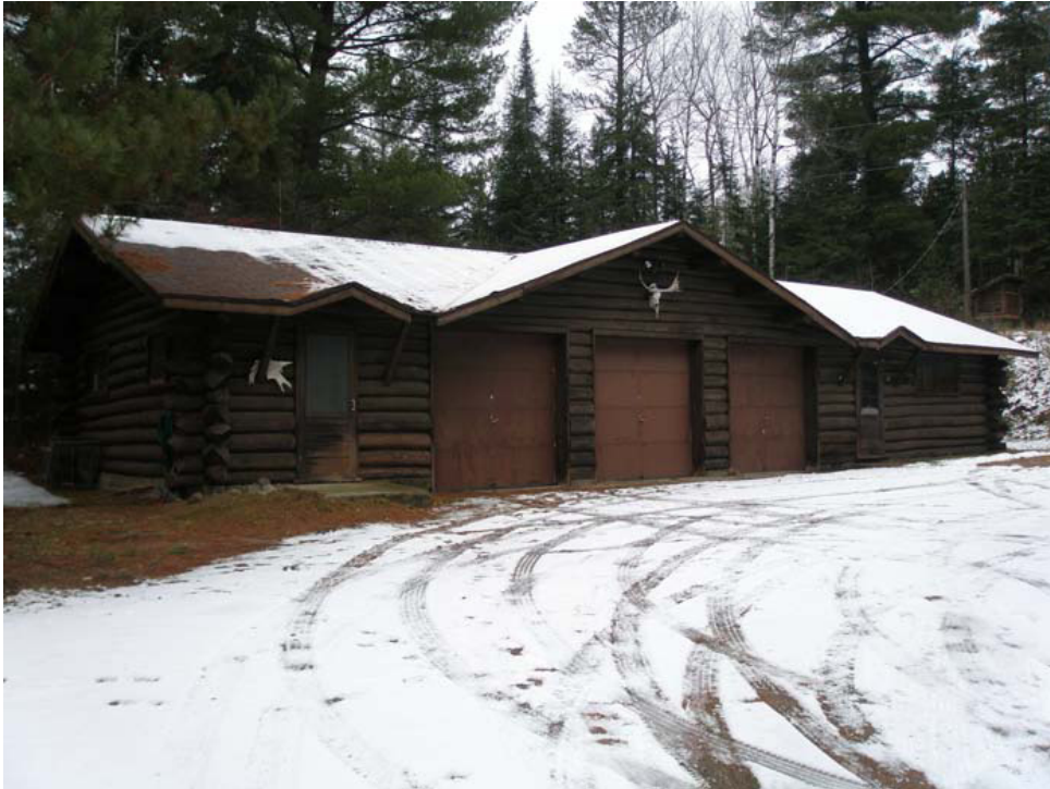
Figure 21. Warehouse/Garage southwest (front) elevation. Note original herring-bone doors have been replaced. (Photo courtesy of Superior National Forest, 2006)
