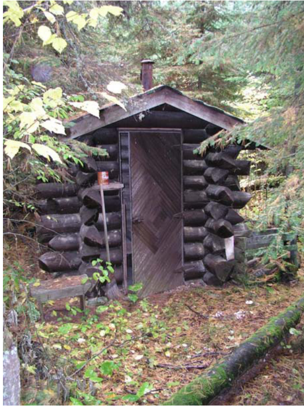
Figure 27. Outhouse, front (south) elevation. Note reoccurrence of diamond pattern door. (Photo courtesy of Superior National Forest, 2006)
