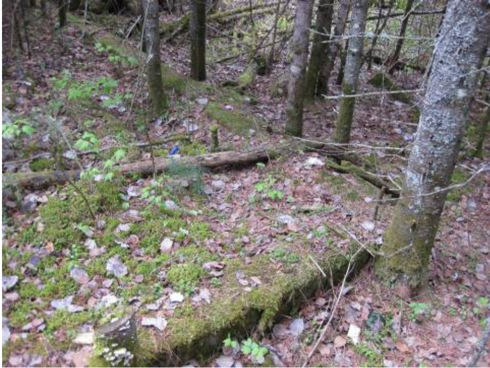
Figure 34. Warehouse foundation (representative of both). (J. Ferguson: June 2, 2009)
