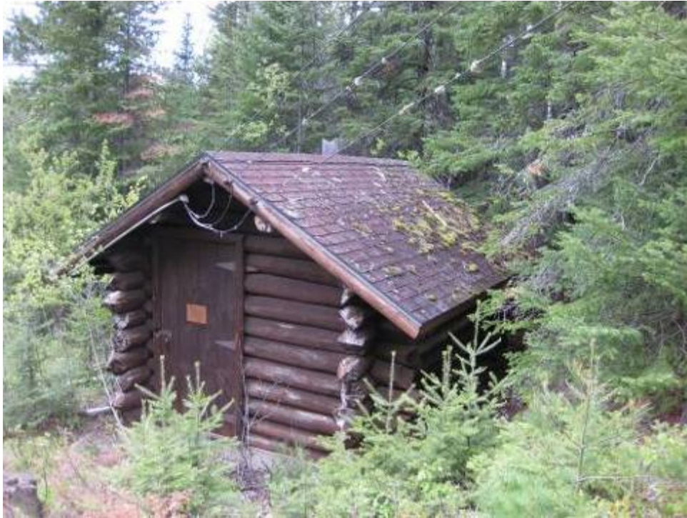
Figure 25. Pump House southwest (front) elevation. (J. Ferguson: June 2, 2009)
