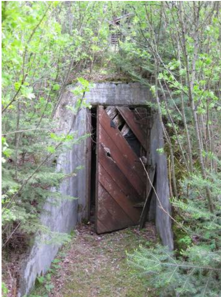
Figure 28. Cellar west elevation. (J. Ferguson: June 2, 2009)
